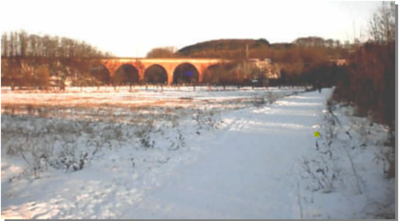
Bogenbrücke in Nidderau—Heldenbergen
